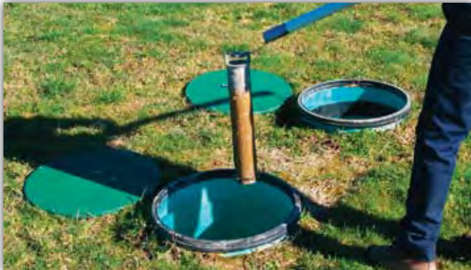
Installing septic risers & lids to your existing septic tank allows access for ease of routine maintenance. Attend a Septics 101 class and you may qualify for a $100 rebate towards installation!
